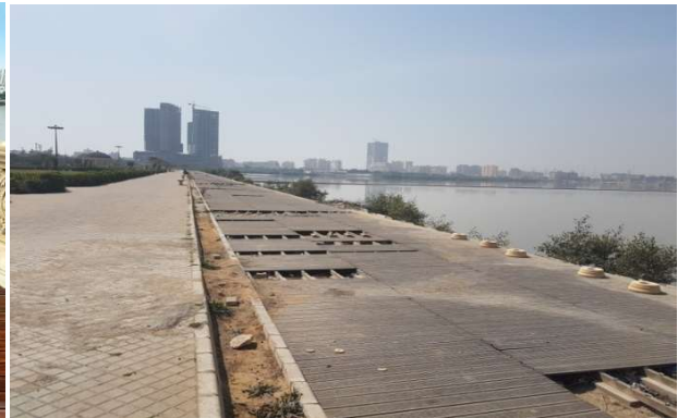
Wooden Board Walkways Condition in 2016
