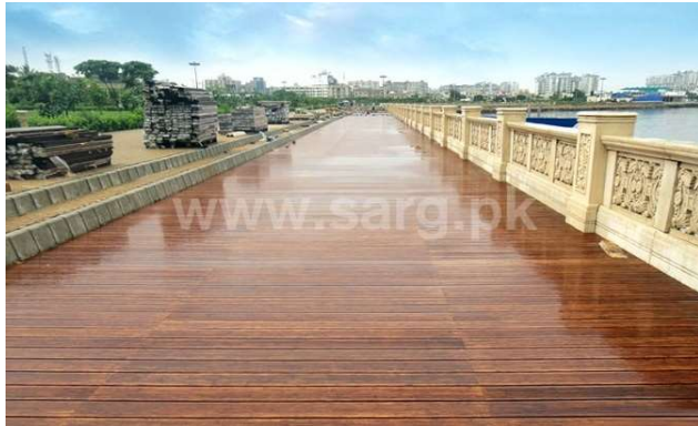
Wooden Board Walk–Condition in 2010
